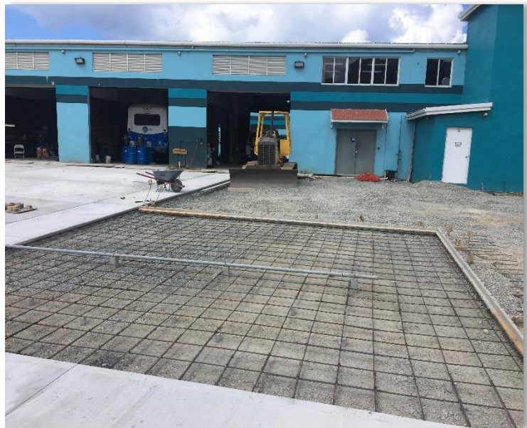
VITRAN Operations & Maintenance Facility – St. Thomas
